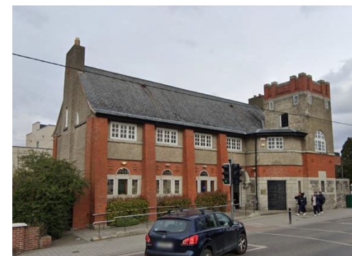
RPS. 149 Public Library, Monastery Road, Clondalkin Two-Storey Library
