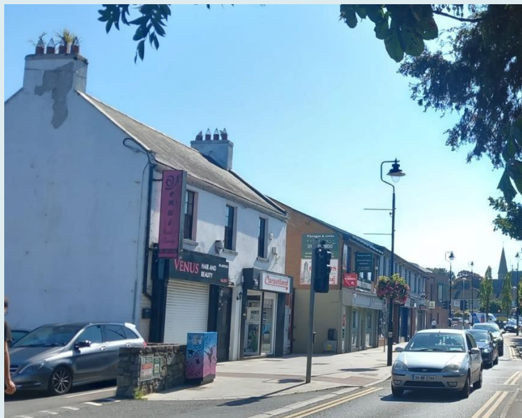
At the southern end of Tower Road, there is a proliferation of oversized plastic signage and external shuttles that detract from the restrained vernacular building forms.
