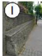
Plinth on Orchard Rd. indicative of line of fosse.
