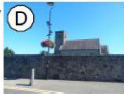
Mixture of random rubble limestone walls and rendered walls on Monastery Rd.
