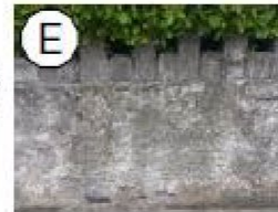
Circa 2.2m high wall, randomly coursed limestone, irregularly shaped blocks with rounded coping.
