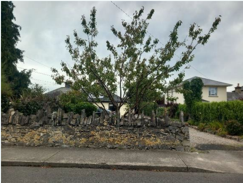
Fieldstone copings in rubble limestone wall, with cut stone defining the openings, Knockmeenagh Road
