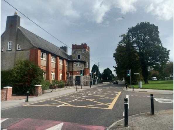
Landmark buildings within the study area create a strong identity and sense of place
