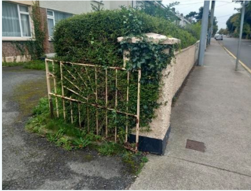
The modest low rendered walls and mid-century Art Deco style starburst gates of mature estates on New Road and Monastery Road sit harmoniously beside the historic limestone walls and create a protective buffer zone around the historic core
