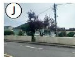
Brick / masonry substrate, with render finish, rounded coping.
