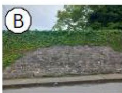
Circa 2.4m high wall, random rubble limestone. Coping excessively weathered / spalled / missing. Extensive washing out of mortar evident.
