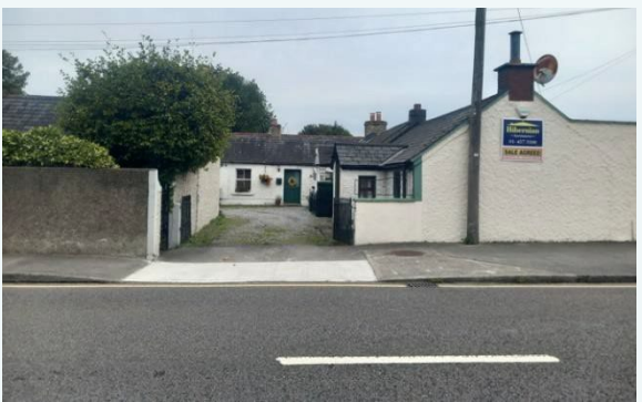
Vernacular buildings forms and limestone walls observed throughout the study area retain the character of an intimate rural village
