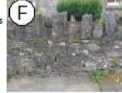
Former Demesne Wall (Floraville House) on Monastery Rd. Rubble limestone, with multiple later interventions
