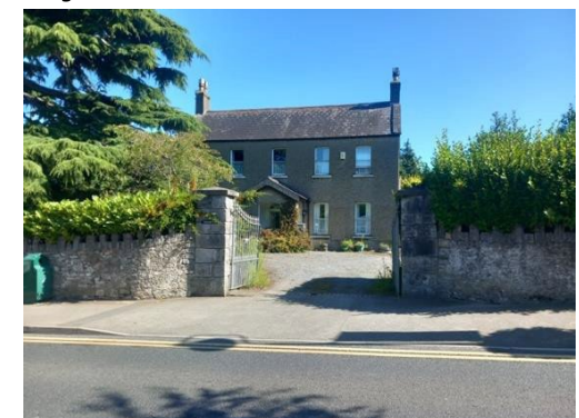
RPS. 419 Towerville, Tower Road, Clondalkin Detached, five bay, two storey house, c.1850
