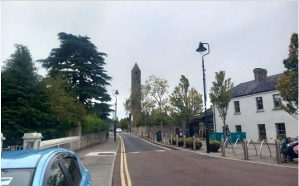
Multiple layers of historic development contribute to the rich tapestry of the village centre
