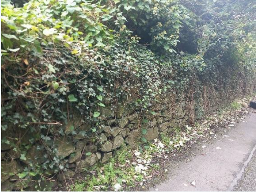
Rubble limestone wall- coping style obscured with overgrowth
