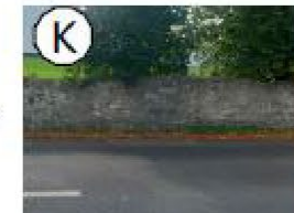
Brick / masonry substrate, with render finish, rounded coping.
