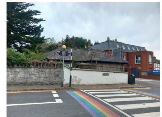
RPS. 153 Convent Road, Clondalkin Detached Multiple Bay Single Storey Former Gate Lodge.
