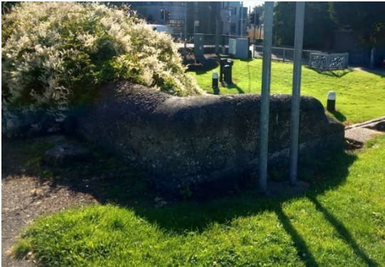
Low walls with half-round coping pertaining to the 19 th century canal infrastructure
